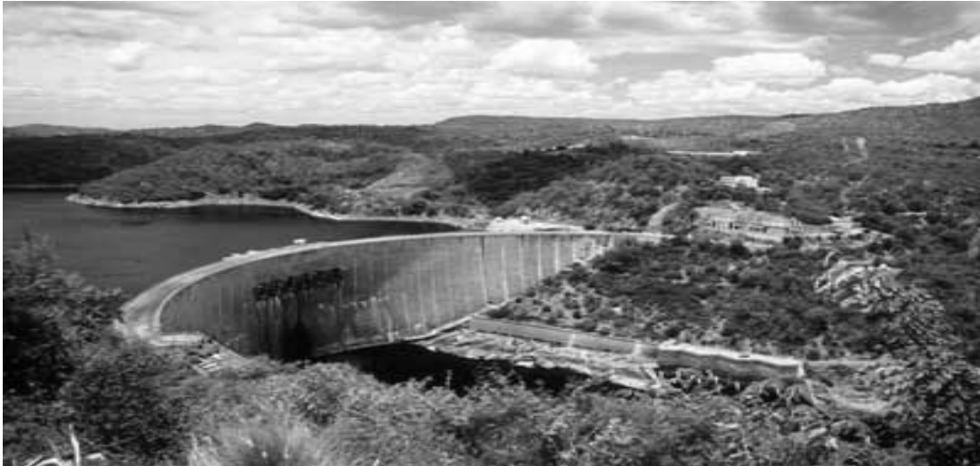
The Kariba dam on the Zambezi river. Part of its function is flood-control
